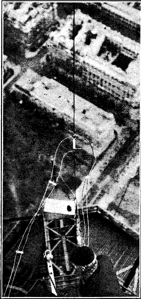
Fig. 1.—The feeder system to one of the aeriels on the summit of the Eiffel Tower is clearly shown in this illustration.
