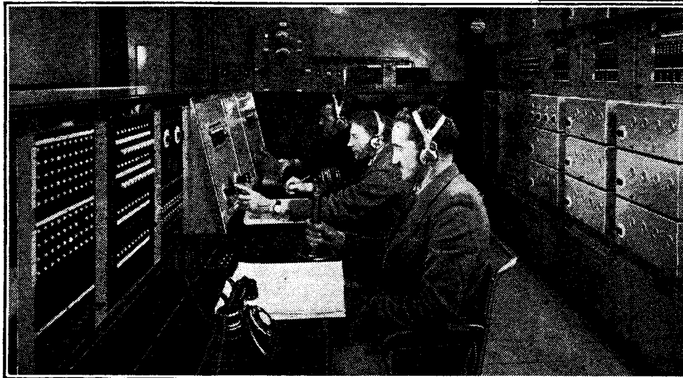
The Bristol Control Room, showing the S.B. and control boards, with the amplifier racks on the right.
